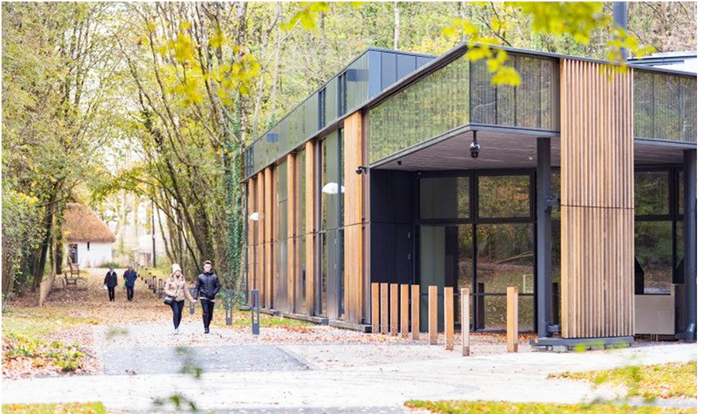
Gweithdy, the new facility for the display, demonstration and practice of crafts and traditional buildings skills at St Fagans National Museum of History ©Amgueddfa Cymru-National Museum Wales.
