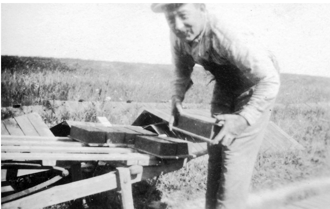
Fig. 6: Here the brickmaker is unloading the newly moulded "green" bricks from the hack barrow at the hack where they are stacked in a long narrow line in layers so as to let the air pass through and slowly dry them. To protect the bricks from the weather, pitched roofing sections made of thin boards called 'Hack Covers' are placed over the top while the drying takes part.
