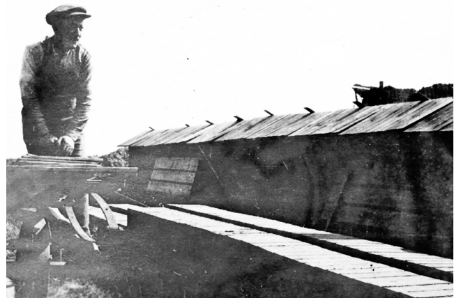
Fig. 7: Although not the clearest photo, the brickmaker is stood with the hack barrow beside a new hack that he is building. Behind the ongoing hack is a completed one with weather protection hack boards sat on top and to the side. After initial drying in the hack the bricks might have been taken to the long, low brick drying shed (Fig. 1) where now dry enough to be stacked in such as herringbone pattern with ventilation breaks, they would remain to finish drying until deemed ready to be fired in the kilns.
