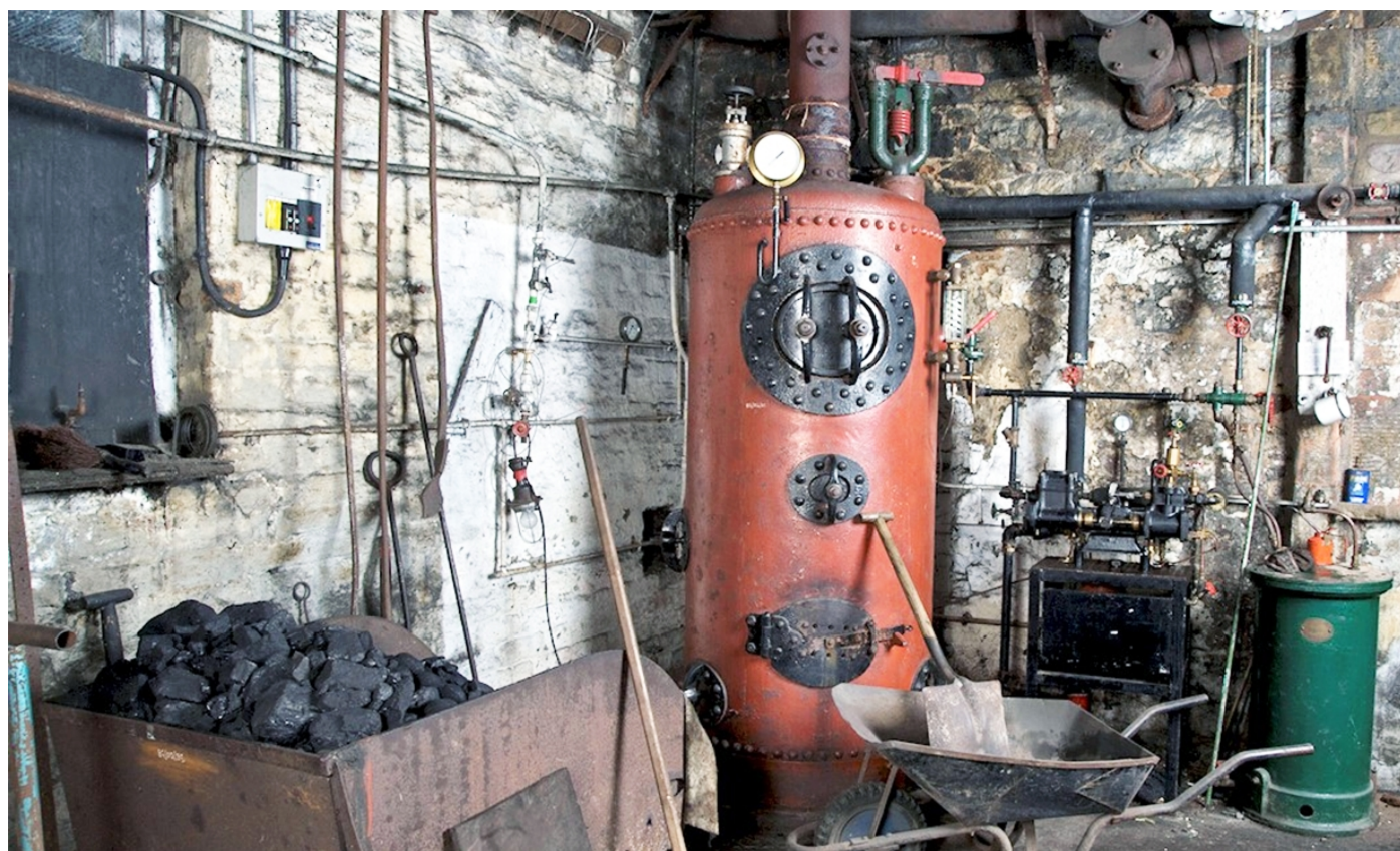
Biggar Gas Works
